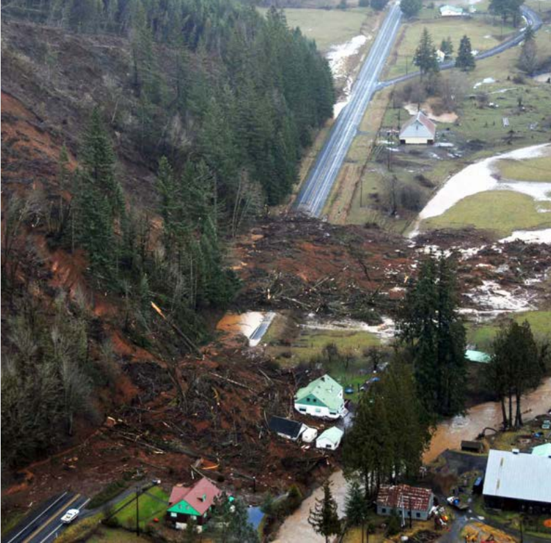
A 2007 landslide caused damage along Washington State Route 6. Washington State Department of Transportation
